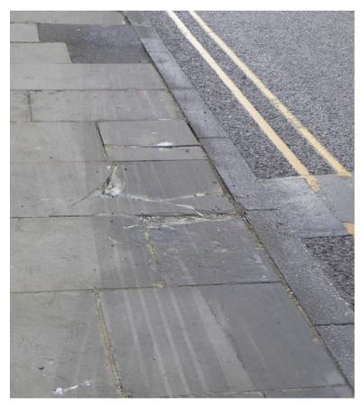
it is because of heavy vehicles turning up the hill from the bus station. I cannot see a simple fix for this simply replacing the flags (whenever that might be) will only be a temporary solution. Perhaps granite stones, similar to those used outside pubs in the old days, are the solution.
